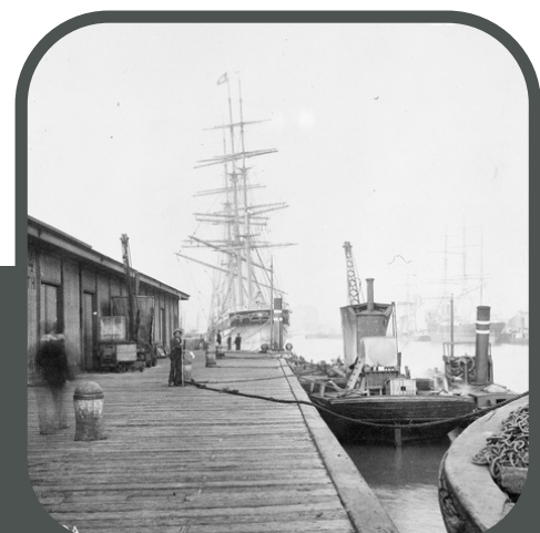
'North Wharf No.14, Melbourne', c.1890, State of Library Victoria, H4417. The large sailing ship is probably docked at No. 12, renumbered No. 5 after 1930. The wharf is constructed from timbers with concrete bollards.
